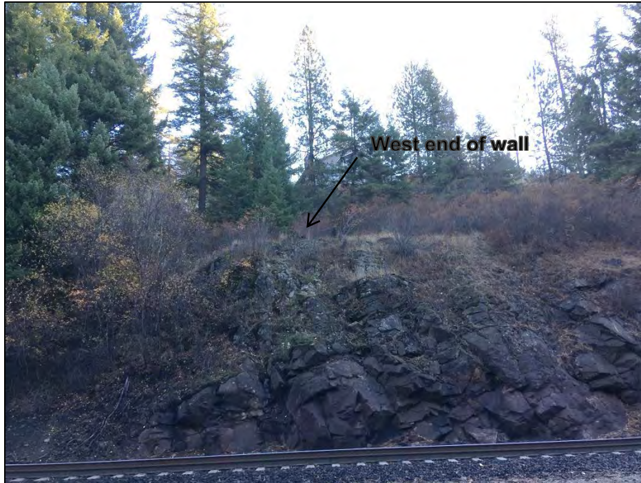
Figure 1. Location of Rock Wall 1 atop rock face; view east from opposite side of railroad.
