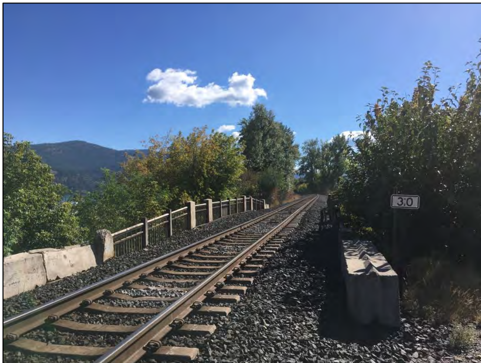
Figure 29. BNSF Bridge 3.1 Railing; View South
