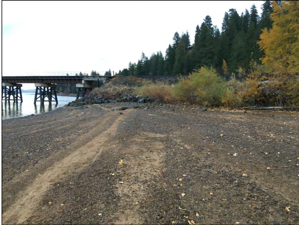
Figure 3. 10BR38 overview below OHWM at Bridge 3.9 south end; view northeast.
