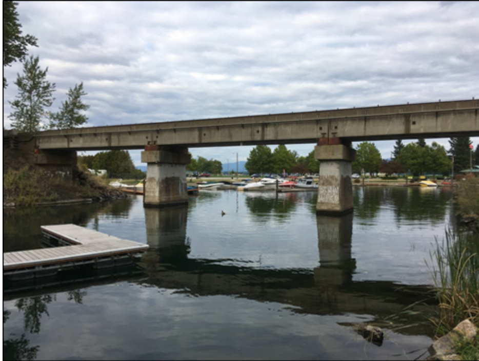
Bridge 3.1, West Elevation
