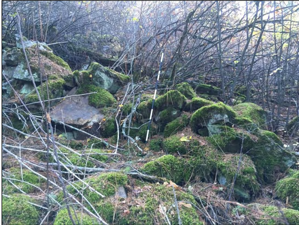
Figure 6. Wall profile near eastern end; view southeast.
