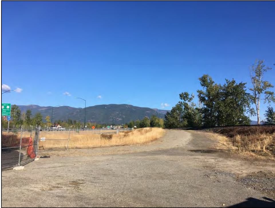
Figure 13. New Fill Prism East of US95, North of Dog Beach; View to North
