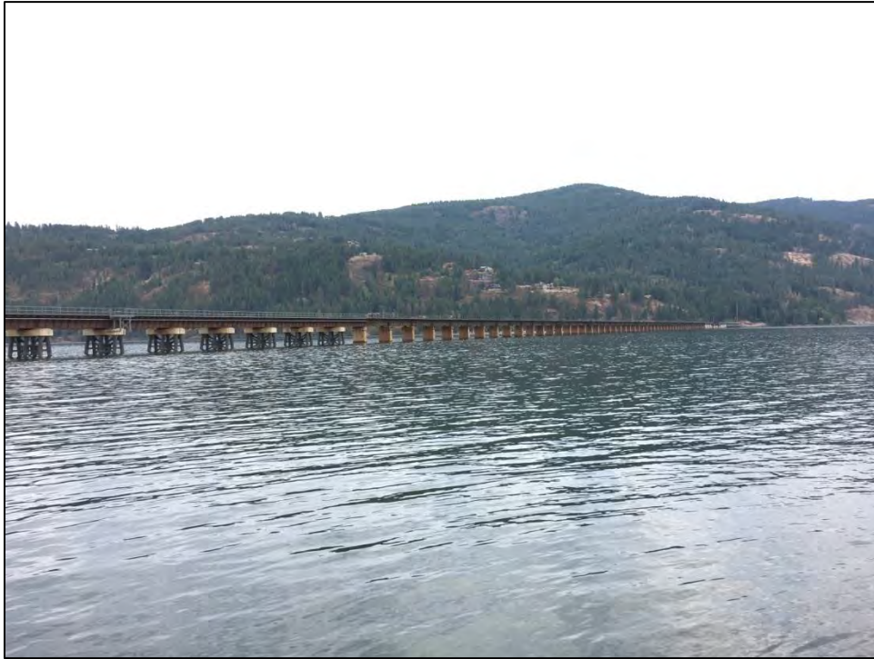
Figure 30. BNSF Bridge 3.9, West Elevation
