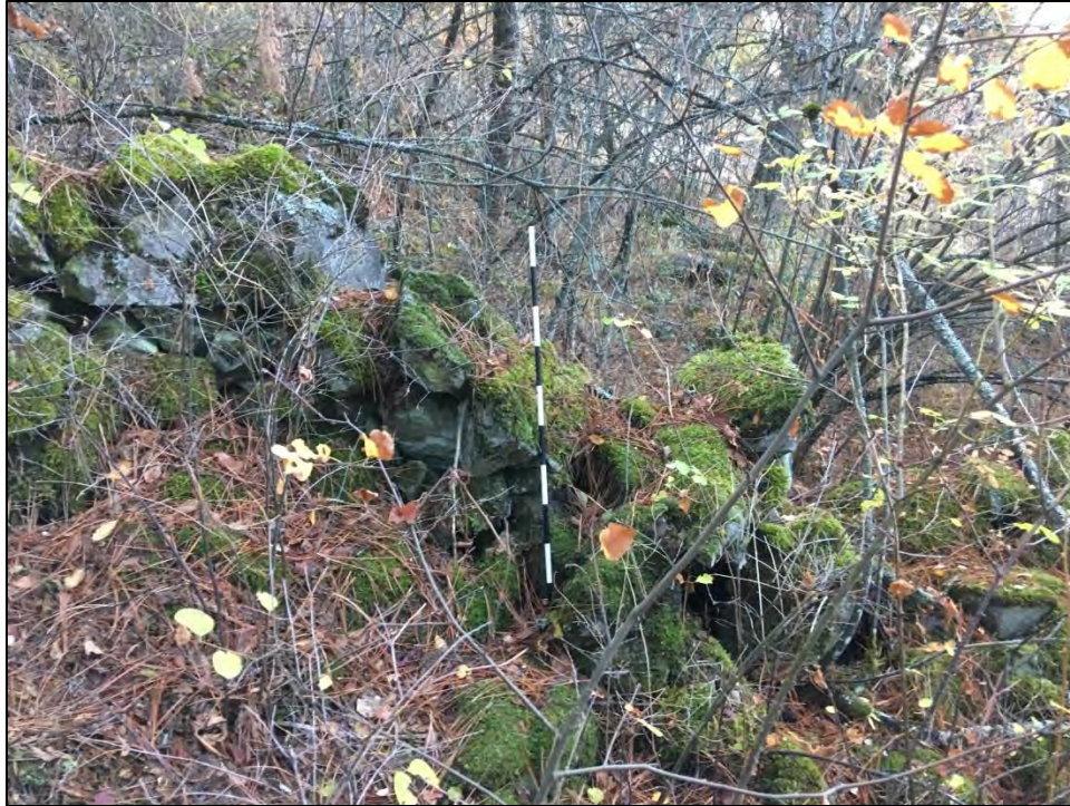
Figure 5. Wall profile on eastern portion; view southwest.
