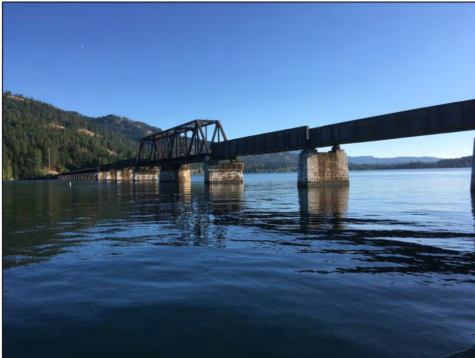
Figure 31. BNSF Bridge 3.9, East Elevation, South Half
